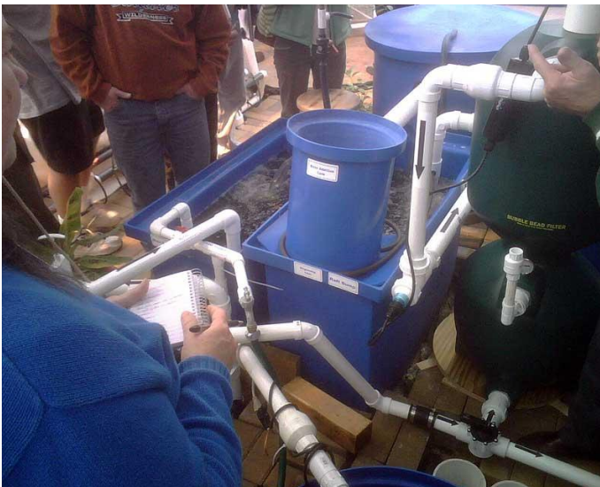
Sump and Base Addition Tank
